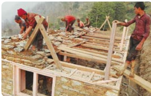
The second level is started
